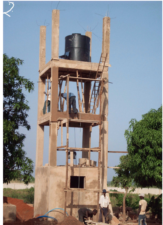
Constructing the Water Tower
